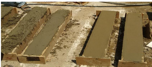
Fig. Casting of beams
