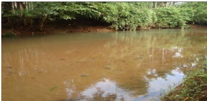
Fig 2. Site for Intake Works at Kottakunnu
